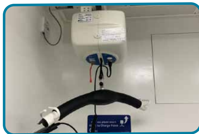
Ceiling track hoist in a CP toilet
