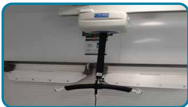
CP toilet with ceiling track hoist
